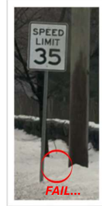
Speed Limit Signs improperly located adjacent to or within 5 feet of utility poles
